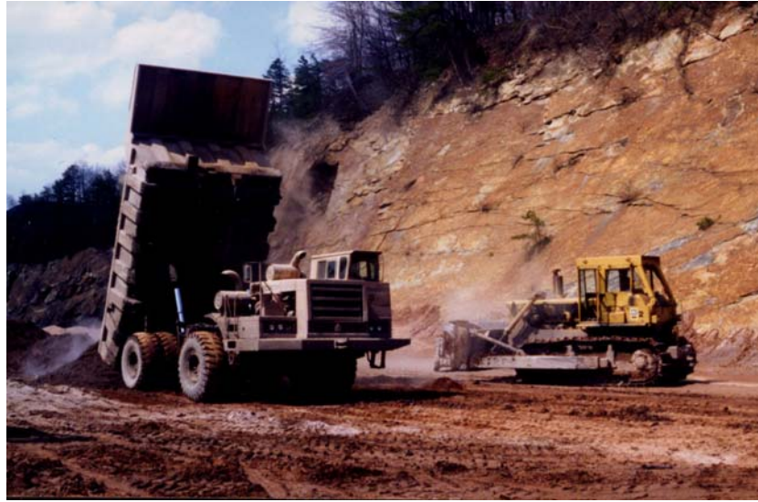
Figure 9.8. A truck and bulldozer used to transport and place ash in the Big Gorilla mine pool.
